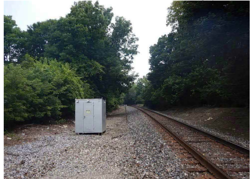
Photo 3. Facing east along railroad from railroad crossing.
